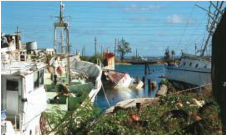
More typhoon damage at the Small Boat Marina and Refuge in Piti.
