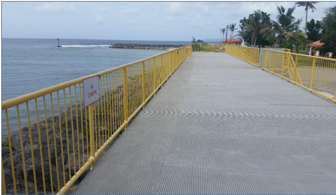
Figure 10: Phase I - Constructed ADA Fishing Platform
