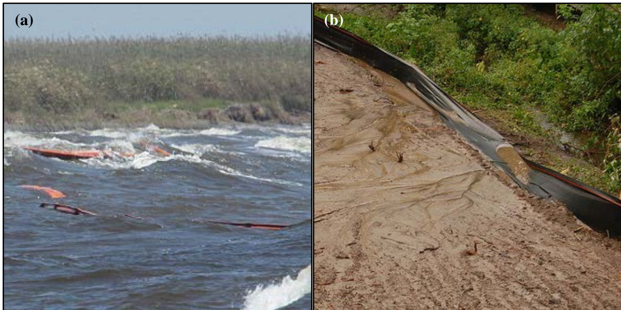
Figure 8. An inappropriately-selected BMP or one that is improperly-implemented is ineffective at reducing the adverse effect of a non-fishing activity on EFH: a) an inappropriately-selected oil control boom for the ocean conditions; b) an improperly-installed silt fence.
