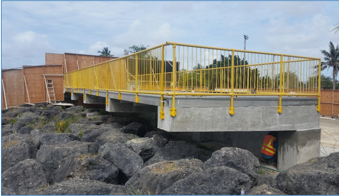
Figure 11: Phase II - ADA Fishing Platform extended 45 ft.
