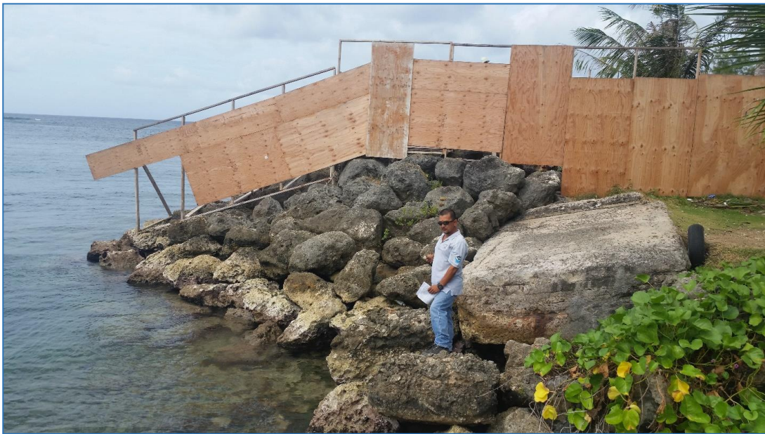
Figure 12: Phase III - ADA Fishing Platform expansion by 45 ft.
