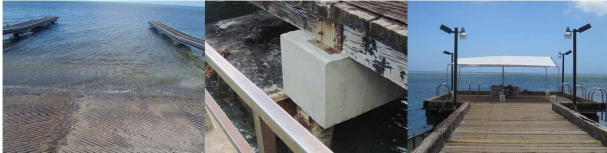
Figure 5. Photographs of Merizo Pier’s repaired walkway and bumpers, concrete support on the pier, and pier lights.
