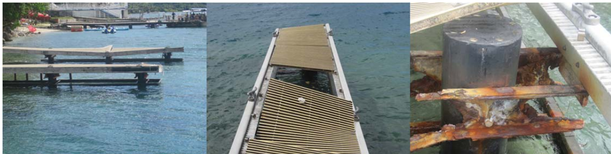
Figure 4. Photographs of Merizo Pier's damaged walkways and bumpers, and rusted walkway pilings.
