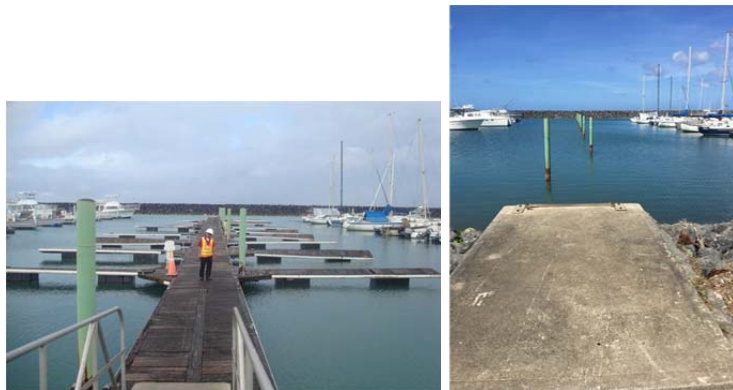
Figure 3. Photographs of Agat Marina's damaged Dock B before and after demolishing using funds from the Department of Agriculture Division of Aquatic and Wildlife Resources' (DAWR) Sport Fish Restoration Program.
