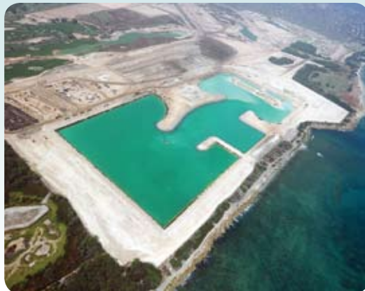
Hoakalei Marina as of June 2008. Photo courtesy of Haseko.
