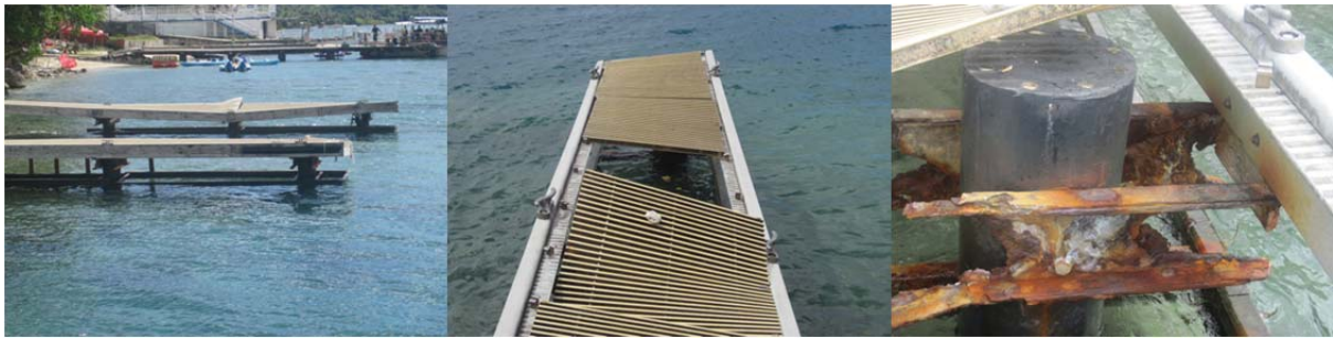
Figure 4. Photographs of Merizo Pier's damaged walkways and bumpers, and rusted walkway pilings.
