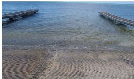
Figure 5. Worn out areas of the boat ramp at Merizo.
