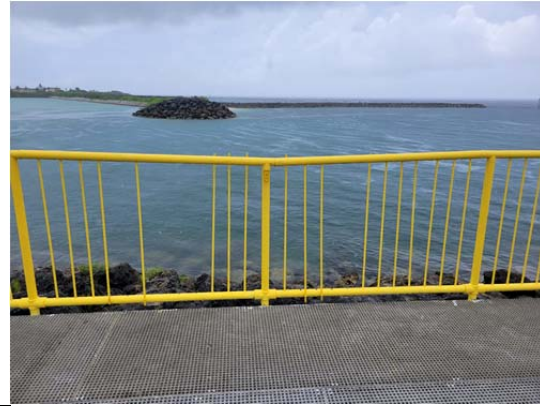
Figure 12. Hagatna fishing platform railings damaged from vandalism after repairs.
