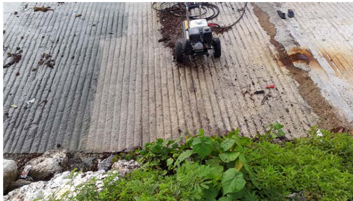
Figure 6: Comparison of the boat ramp after water blasting removed accumulated algae.
