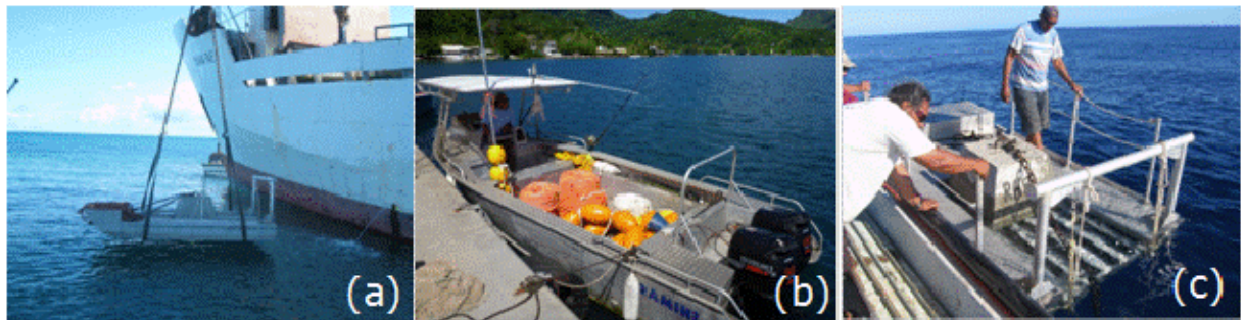
Figure 21. deployment in remote island situation using a portable pontoon barge that supports the FAD anchor.
