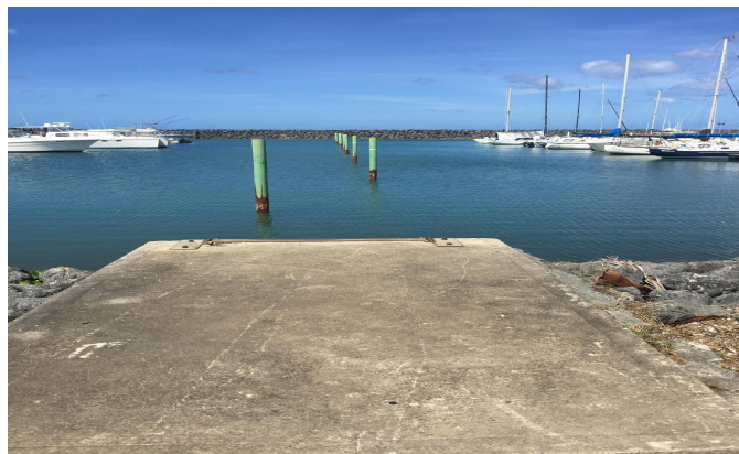
Figure 2. Site of Dock B with damaged decking removed.
