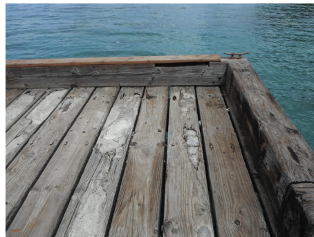
Figure 4. Damaged pier walkway planks temporarily filled with concrete to reduce additional plank damage by wood rot.
