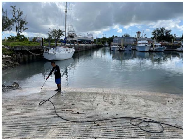
Figure 4: Fisheries staff water blasting the back ramp at the Agana Boat Basin.
