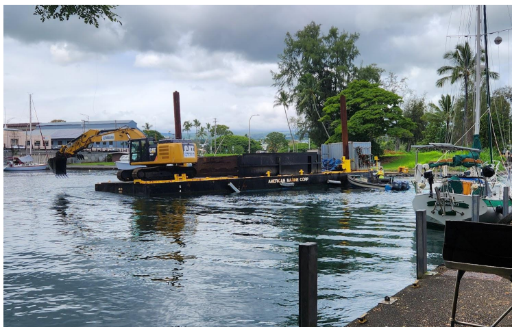
Dredging of Hilo Harbor channel.
